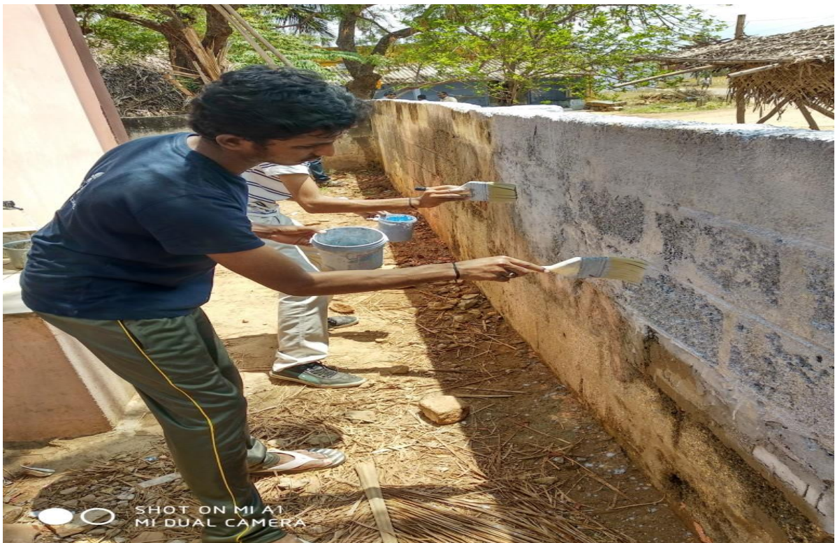
Our NSS Volunteers Repainting the School Compound Walls, School Walls and Kitchen Rooms
