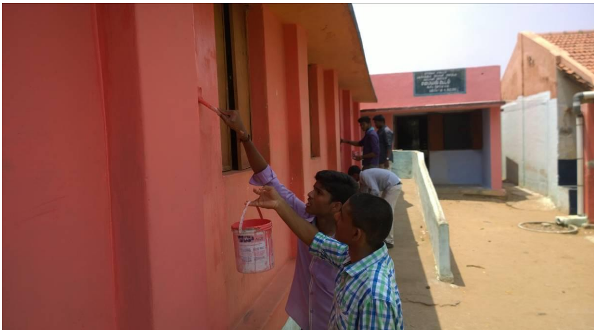
NSS Volunteers Repainting the School Walls. (16.04.2016)
