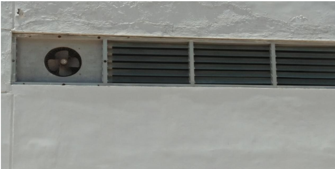
Fig.4. Exhaust fan located in the toilets
