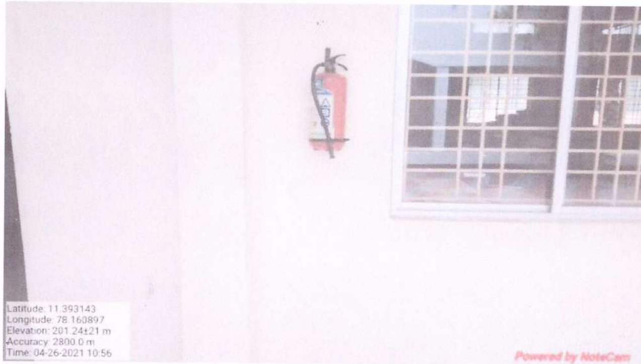
FIRE EXTINGUISHER NEAR CAD/CAM LAB
