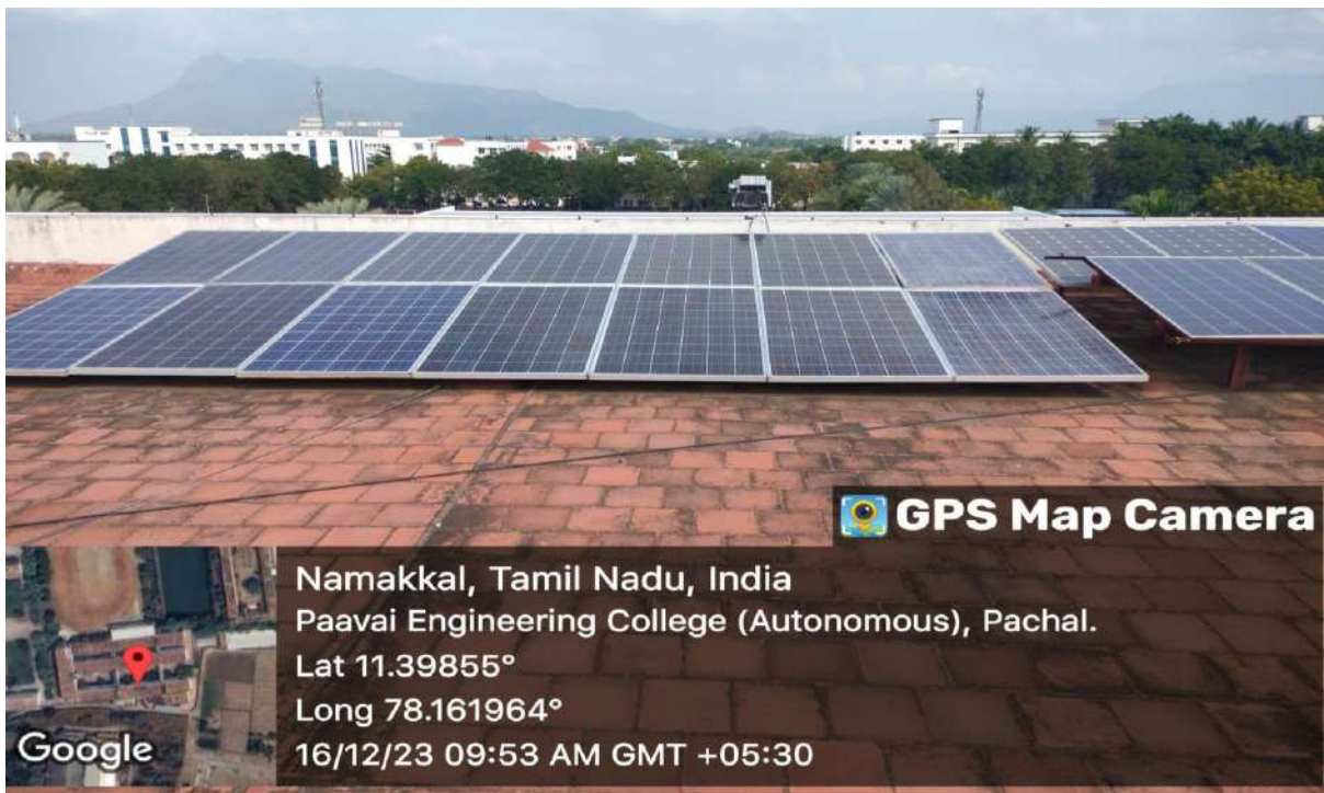
Fig: Solar control Panel
