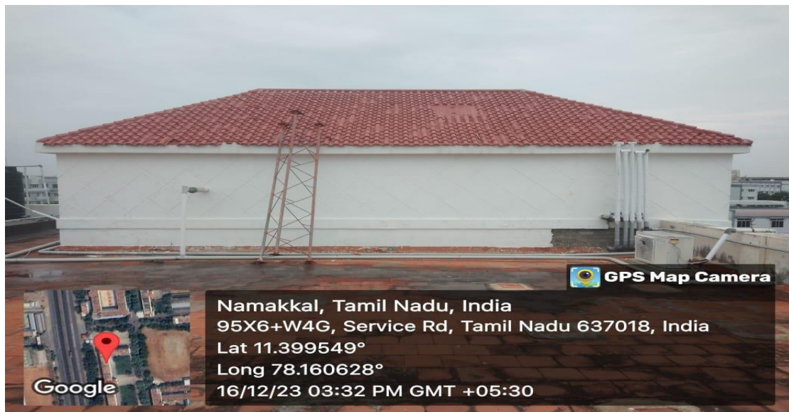
Water Tank 1 with capacity of 6,000 Litres
