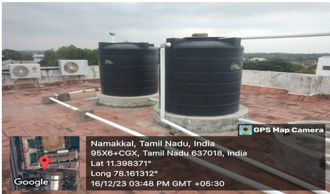
Water Tank 4 with capacity of 2,000 Litres each
