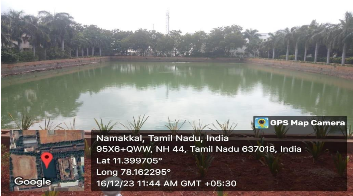
Rain Water Harvesting: Capacity 2 Crore Litres
