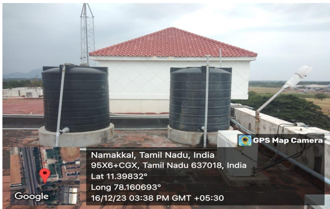
Water Tank 5 with capacity of 2,000 Litres each
