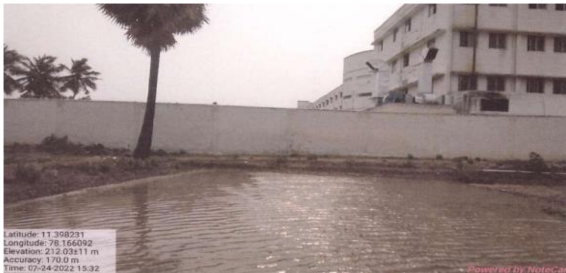
Construction of Bunds
