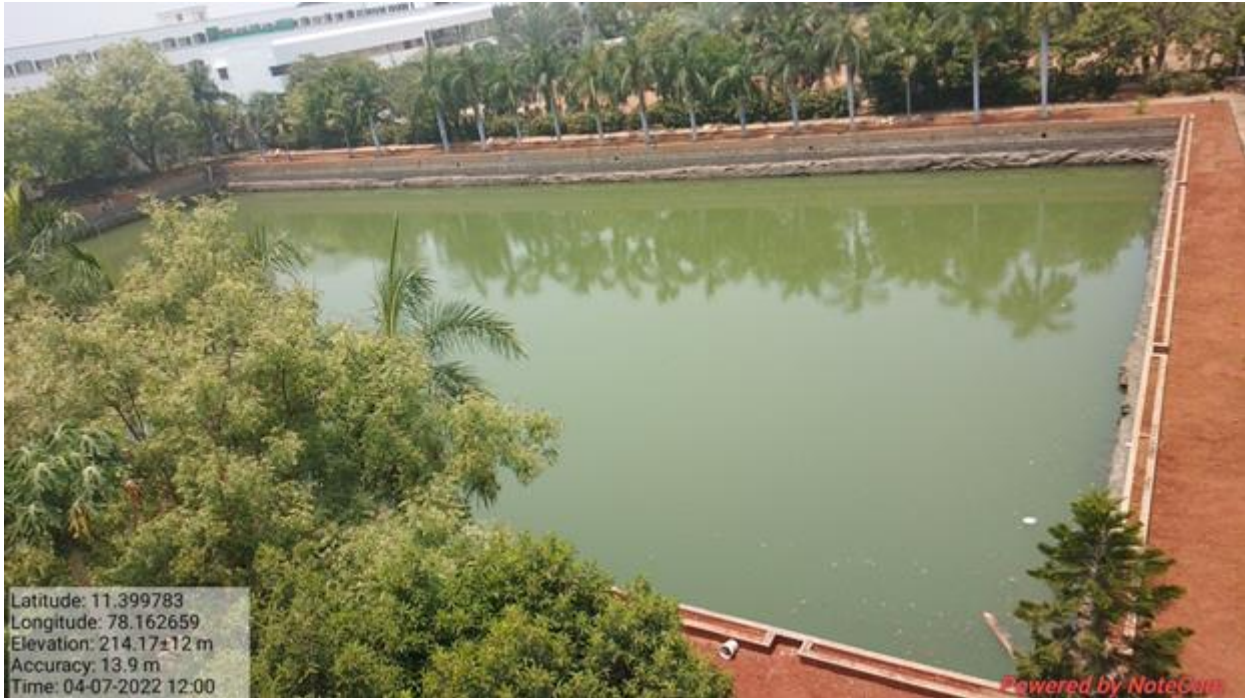
‘AMIRTHAVARSHINI’ a Mega Rain water Harvester
