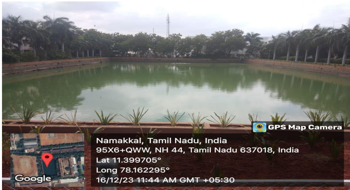
‘AMIRTHAVARSHINI’ a Mega Rain water Harvester
