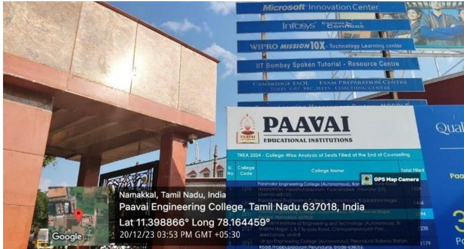
CCTV CAMERA IN MAIN ENTRANCE GATE
