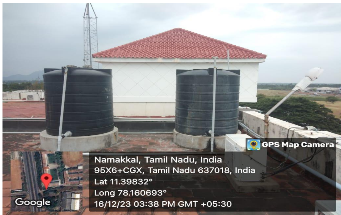
Water Tank 5 with capacity of 2,000 Litres each
