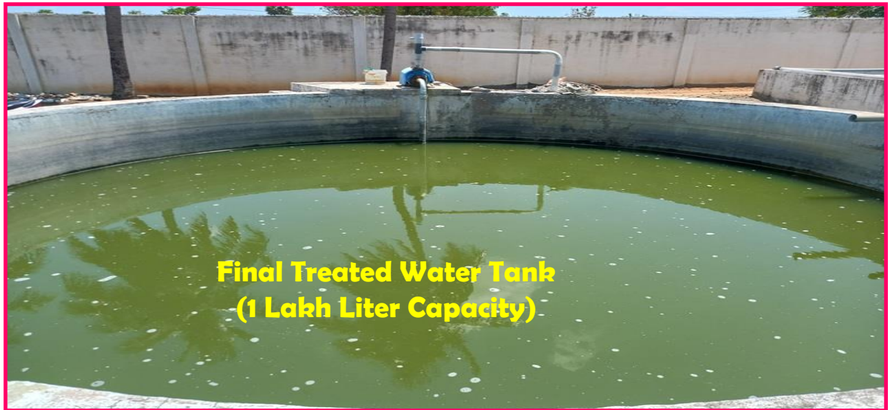
Various Stage of Sewage Treatment Plant (STP)
